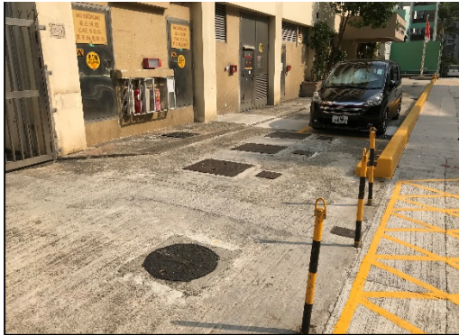
Hack-off and cart away the existing concrete kerb and install new chained stainless steel bollard posts
